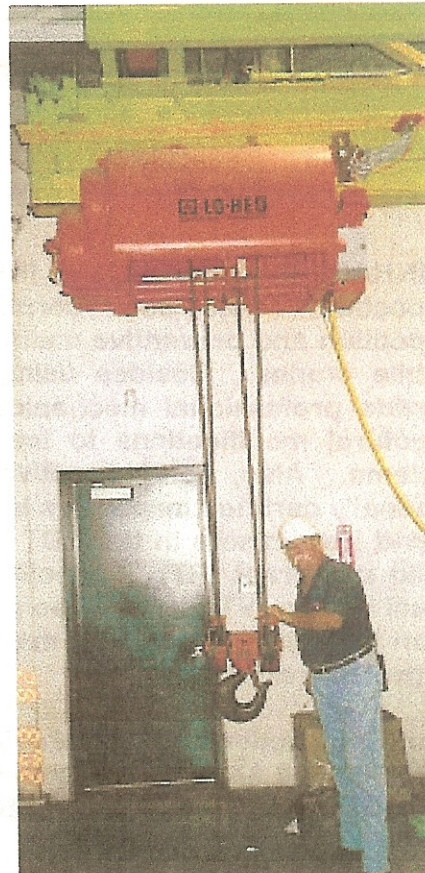
Inspection of 10-ton crane
